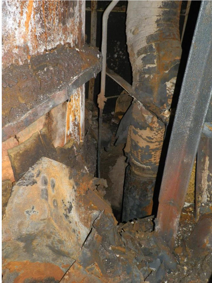
Figure 9: Capture of the inside of the port funnel duct
