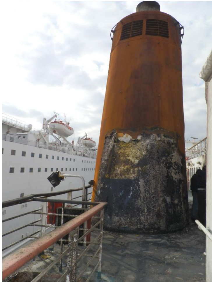
Figure 5: Capture of the fore side of the port funnel duct
