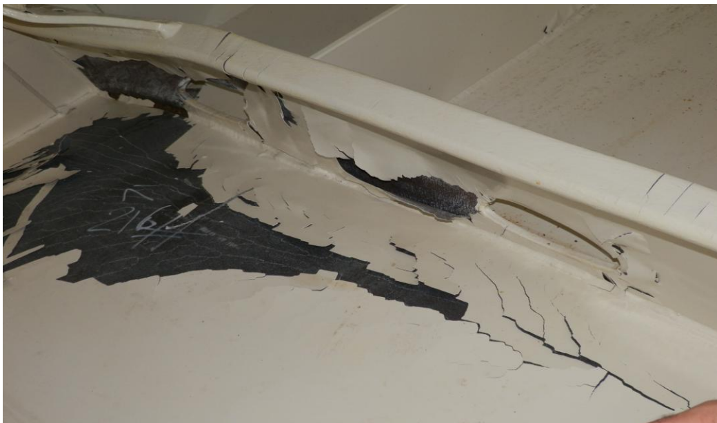
Figure 32. The indents sustained on the hull plating under the waterline caused by the contact on the breakwater substructure.
