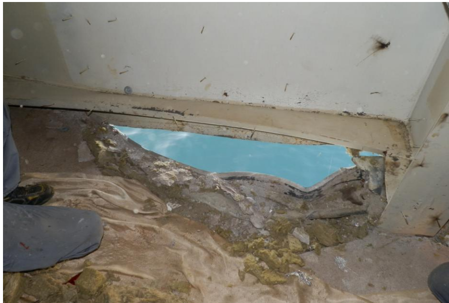
Figure 29. The sustained crack from inner view caused by the impact on the head of the breakwater.
