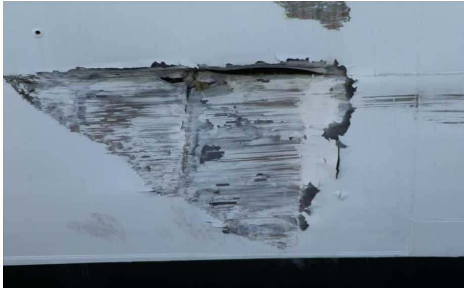
Figure 28. The sustained deformation and crack to hull caused by the impact on the head of the breakwater
