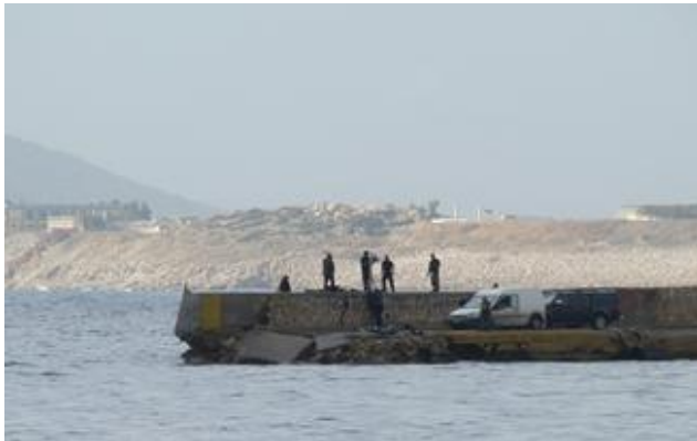
Figure 2: The damaged head of the breakwater.
