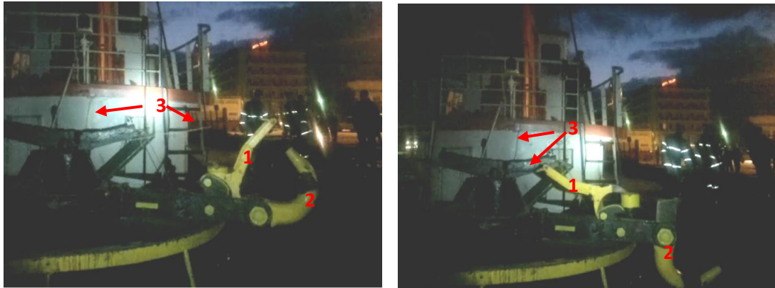
Picture 3: Arrangement of the quick release mechanism of ARTEMIS V. The releasing phases prior to activation (on the left) and past activation (on the right). 1: Hook fastening arm, 2: Towing hook, 3: Release wire from the coupled jointed arm to the bridge.
