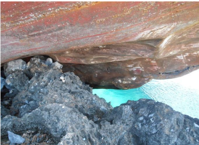
Deformed starboard bottom fore section.
