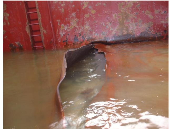
The crack at inner bottom plate of No 1 cargo hold.
