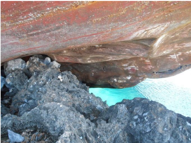
Deformed starboard fore bottom section.
