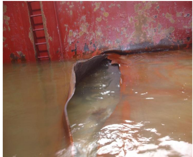
The crack at inner bottom plate of No 1 cargo hold.
