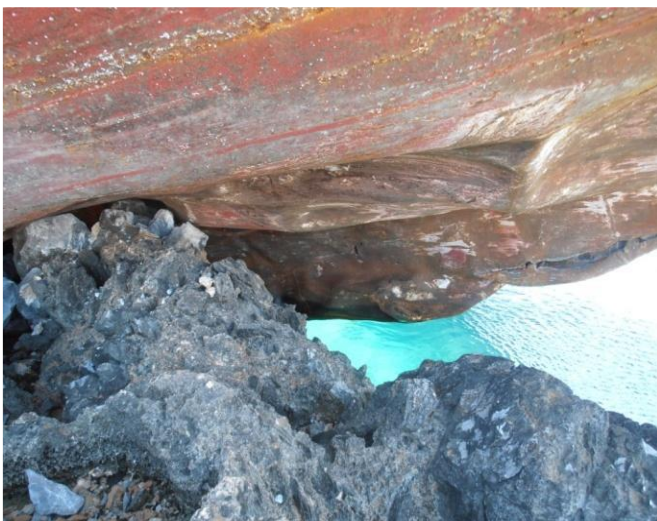
Deformed starboard bottom fore section.
